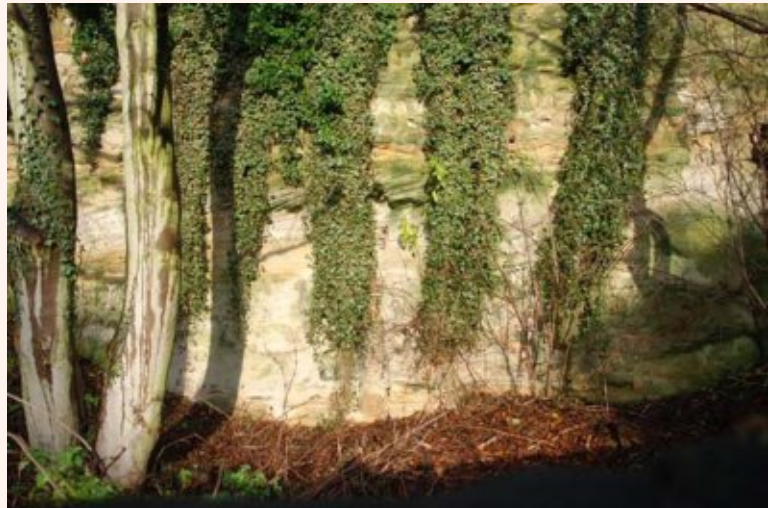
Thorner Quarry - before vegetation removal
